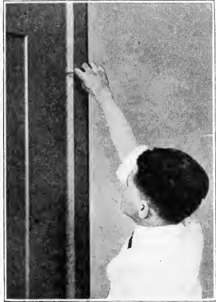
FIG. 448. MARKING DOOR AND FRAME FOR HINGE LOCATION.
